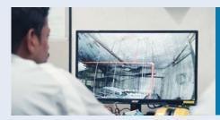
At Tiong Bahru Plaza, a CCTV camera in the chiller plant room provided a safer way to monitor water seepage, reducing the need to work at heights. To further improve electrical safety in the chiller plant room, the team added an acrylic screen between the pumps and electrical boards, protecting the boards from potential water exposure in the event of a leak.
