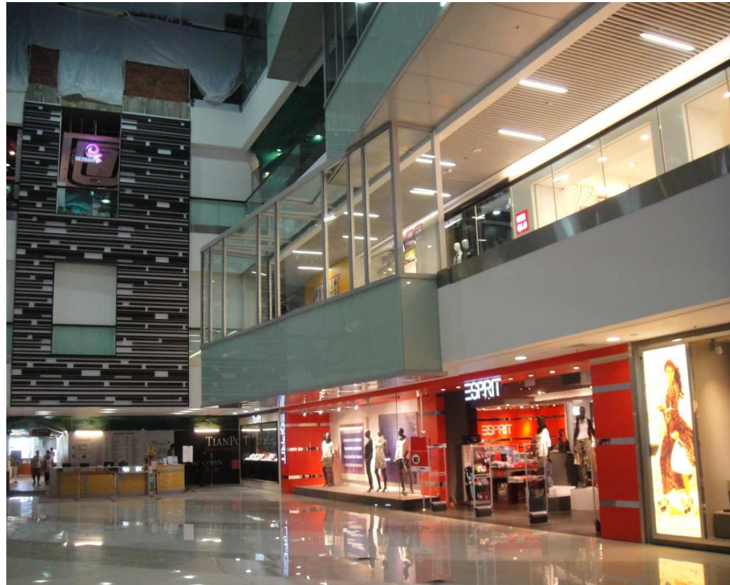
Completed works at Level 1
