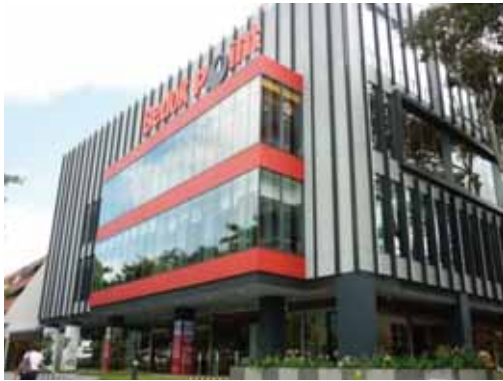
PICTURE 1 – BEDOK POINT, EXTERNAL VIEW
