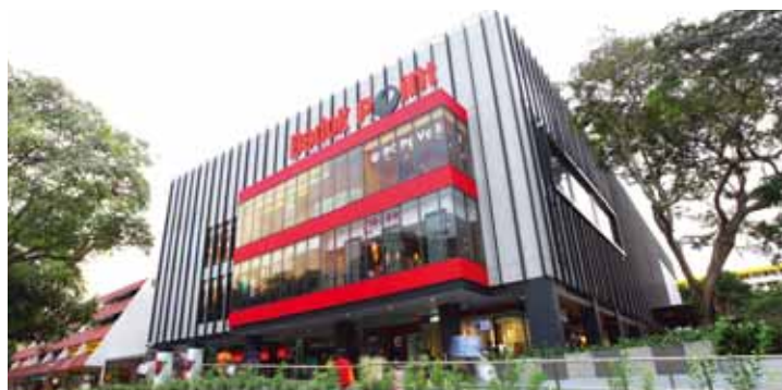
Exterior view of Bedok Point
