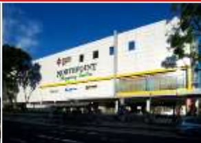
Northpoint City North Wing + Yishun 10 Retail Podium
