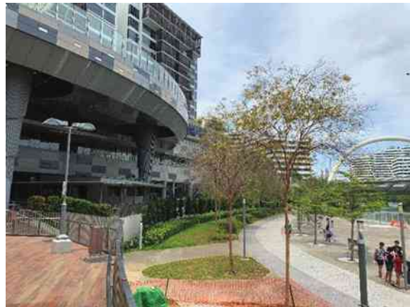
Picture 6 – Frontage to My Waterway @ Punggol
