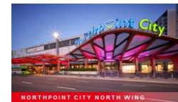
NORTHPOINT CITY NORTH WING
