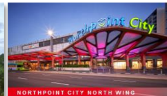
NORTHPOINT CITY NORTH WING
