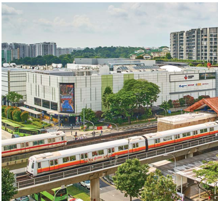
Northpoint City North Wing, Singapore
