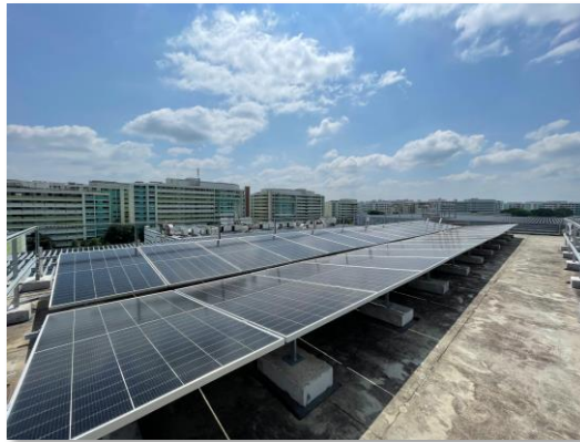
Northpoint City North Wing
